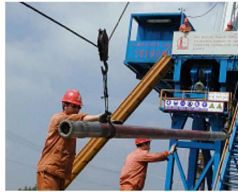
Figure 2: The Workers Use the Pneumatic Winch Steel Wire Rope and Hook
