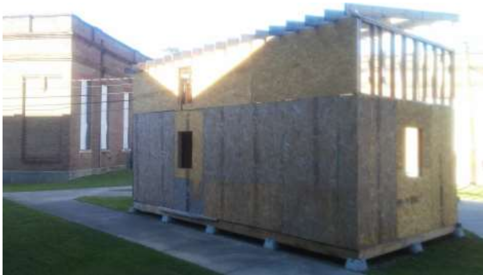
Figure 1: Tiny house at the beginning stages before getting finished. The wall is still fitted with rough lumber sheathings laid on studs and sole/double plates.
