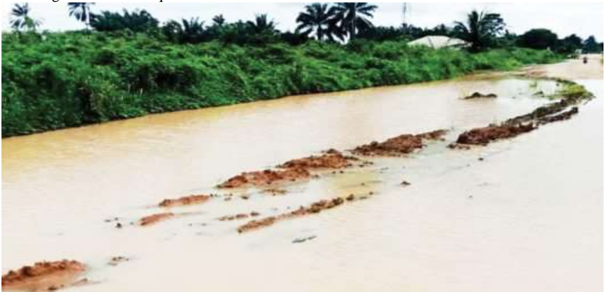
Fig.3. Submergence effect on topsoil foundation in Eket
