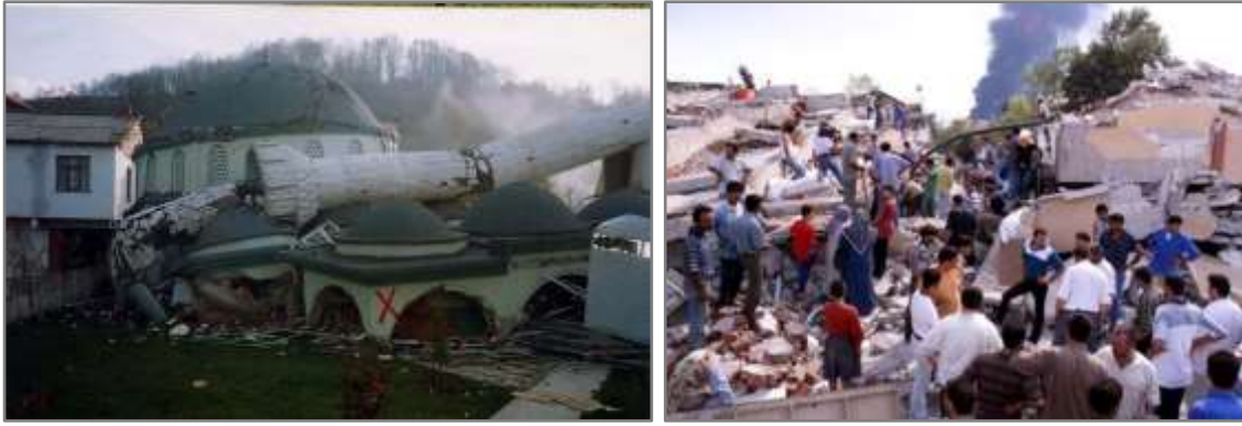
Figure 1: Example of damage caused by an earthquake (Parsa, 1999)
