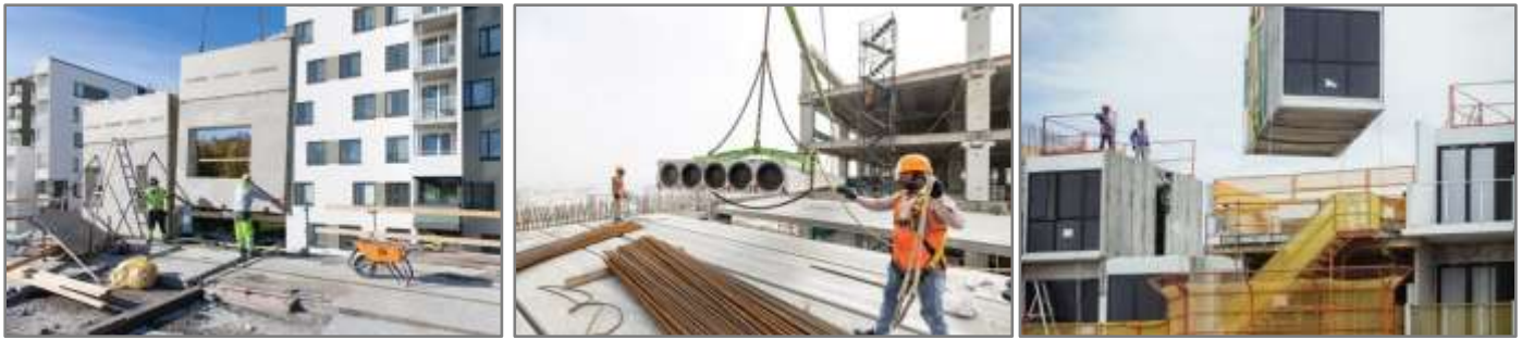
Figure 3: Precast concrete systems (a) Frame system, (b) Panel system, (c) Cell system (URL-1) (URL-2)
