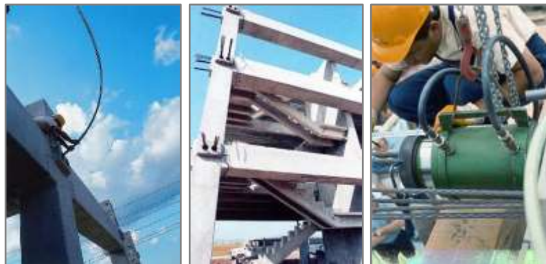
Figure 4: Post-tensioning steps (URL-3)
