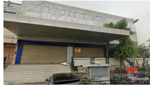
Figure 2 Empty Building Former Hypermart Modern Market
