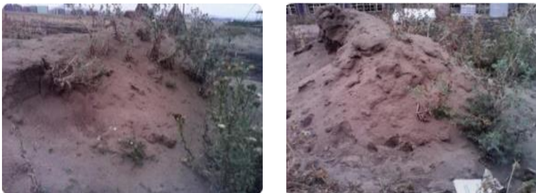
Figure 4.4: Poor handling of fine aggregates (sand) on construction sites Jasikan Source: Field research
