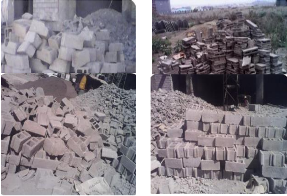
Figure 4.1: Wastage of CHB on building construction sites due to poor handling at Ho-Poly. Source: Field research
