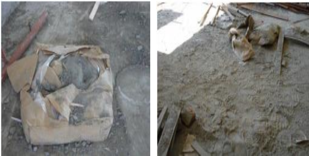
Figure 4.7: Wastage of cement due to poor handling, Lack of control & poor storage Source: Field research
