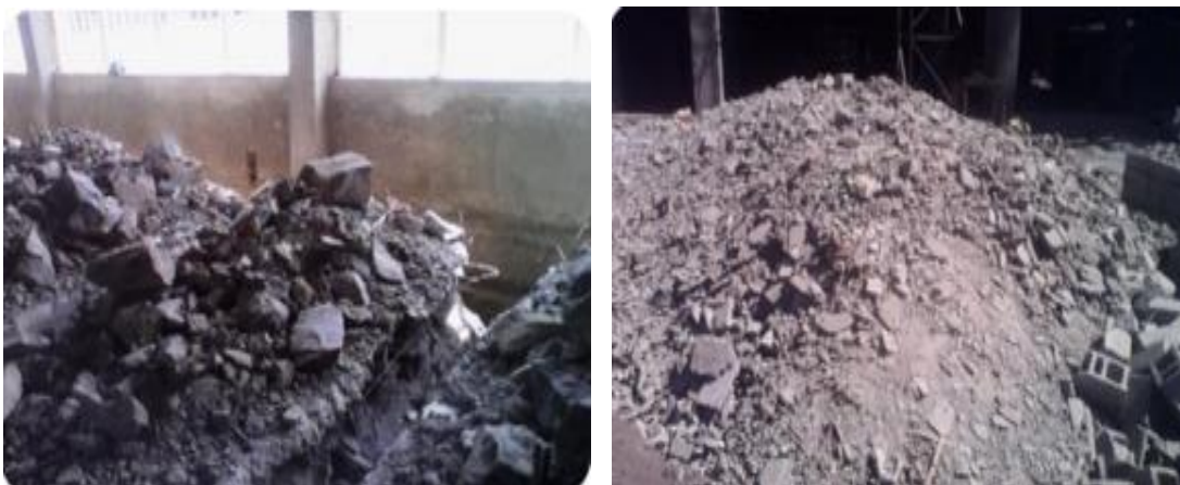
Figure 4.8: Wastage of cement mortar due to chiseling & design change on building Sites. Source: Field research
