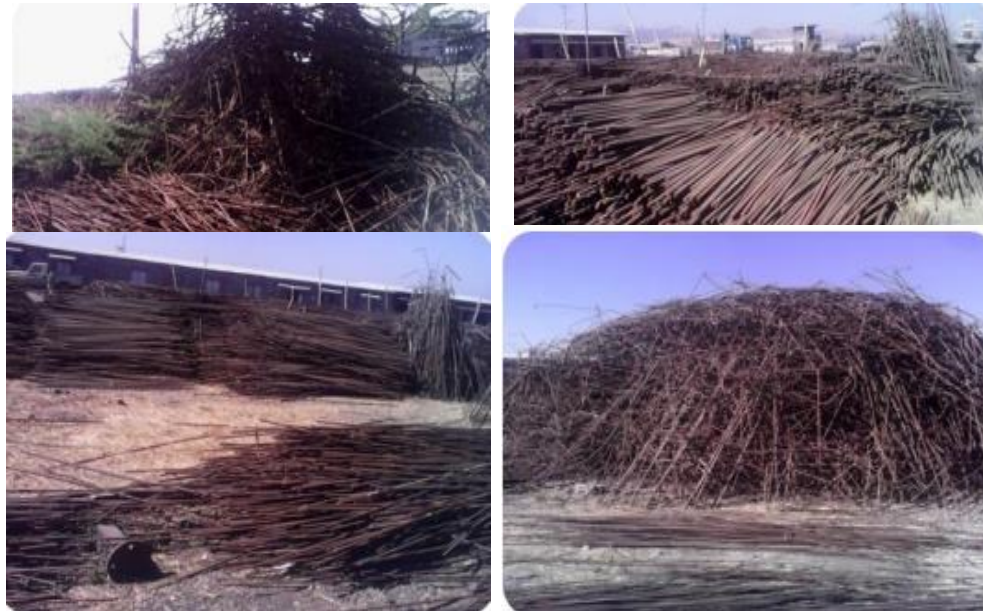
Figure 4.3: wastage of steel reinforcement bar due to Non- optimized cutting of bars and design change. Source: Field research
