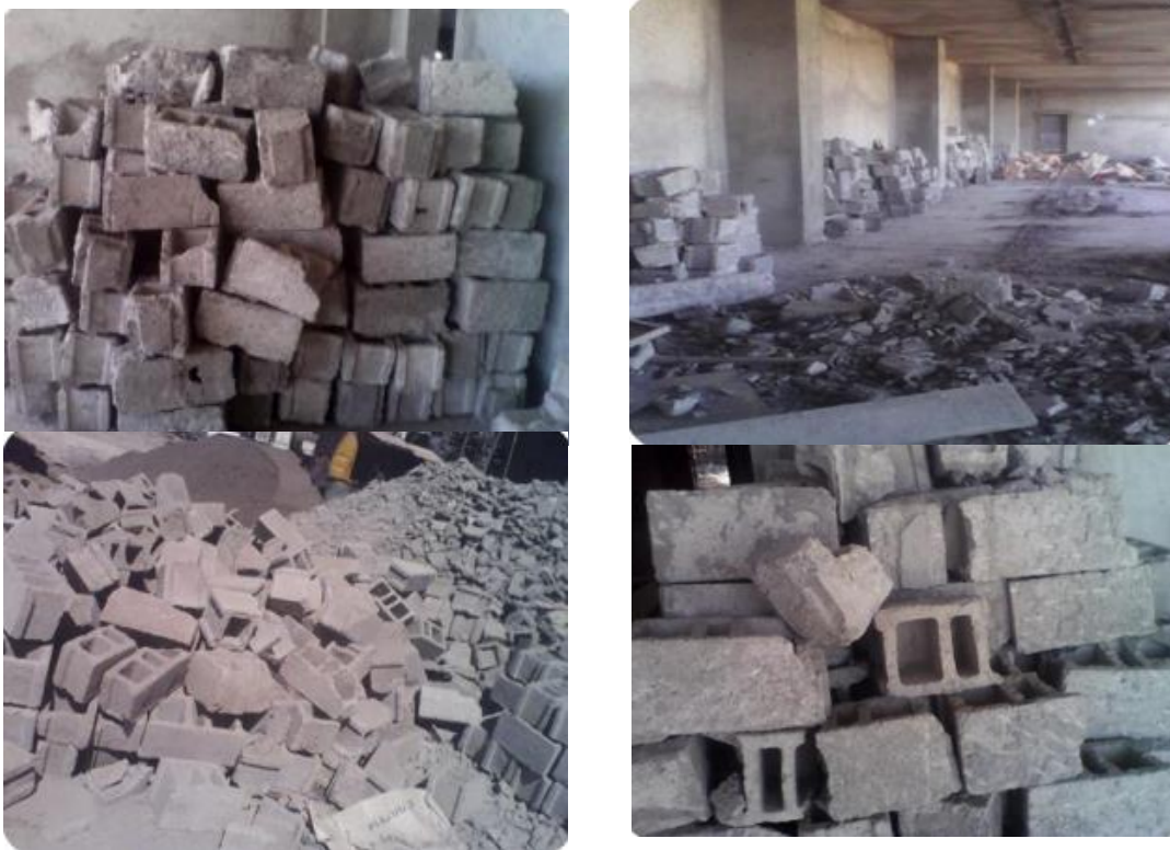
Figure 4.2: Wastage of HCB on building construction sites due to change orders at Ho-Poly. Source: Field research
