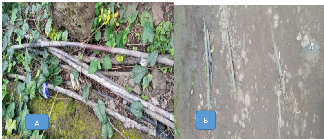
Plate 1: The placement of water distribution pipes in Molyko
